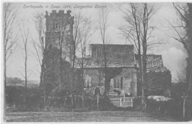
Postcard showing damage to Langenhoe church following the earthquake.
